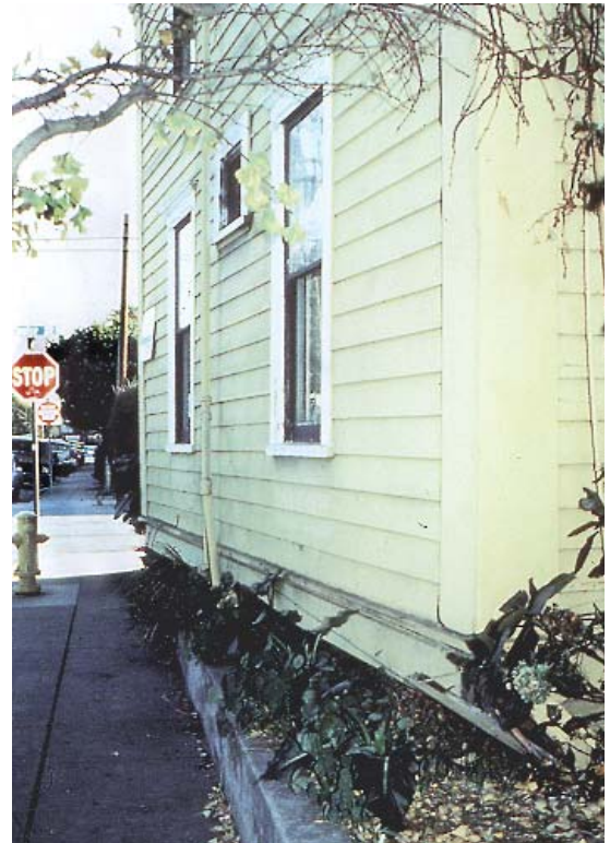
Cripple wall foundation failure, Northridge, Calif.
