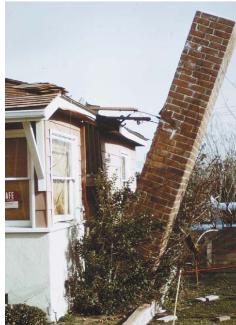
Chimney damage, San Fernando, Calif.
