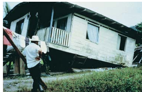
Post-and-Pier Foundation; undamaged (top) and damaged (bottom), Costa Rica.
